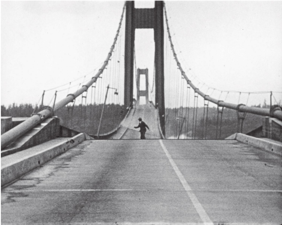
FIGURE 9.2. The Tacoma Narrows Bridge, moving like a bullwhip as it collapsed. (Photo courtesy of University of Washington, University Libraries Special Collections, UW20731.)
